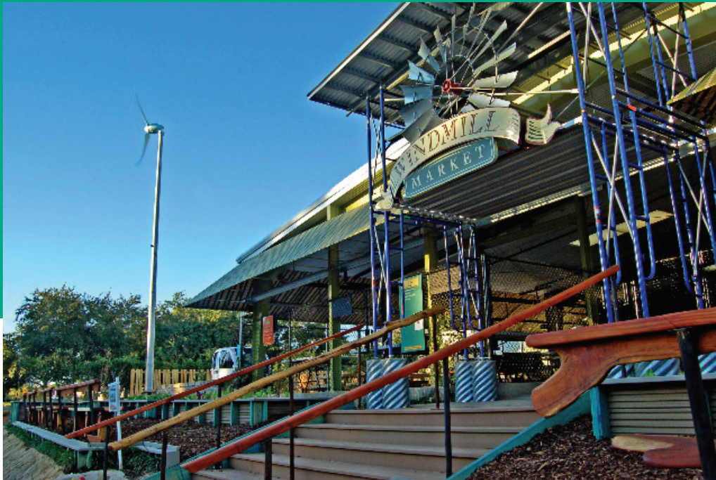
Lively graphics, a deep-awning and bright details turned a forlorn metal building into Windmill Market. The modern windmill generates power.
