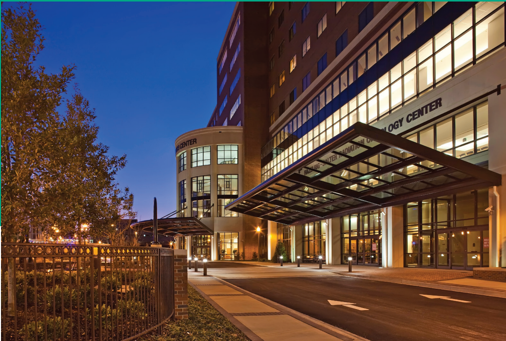
A projecting rotunda marks the entrance to UAB's new Women & Infants Center. Entrance to the radiation oncology center is on the right.
