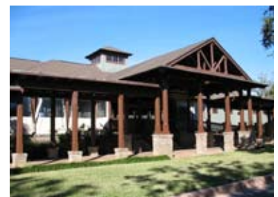
Chamfered wood columns raised on brick piers repeat an architectural detail found on many Point Clear porches.
